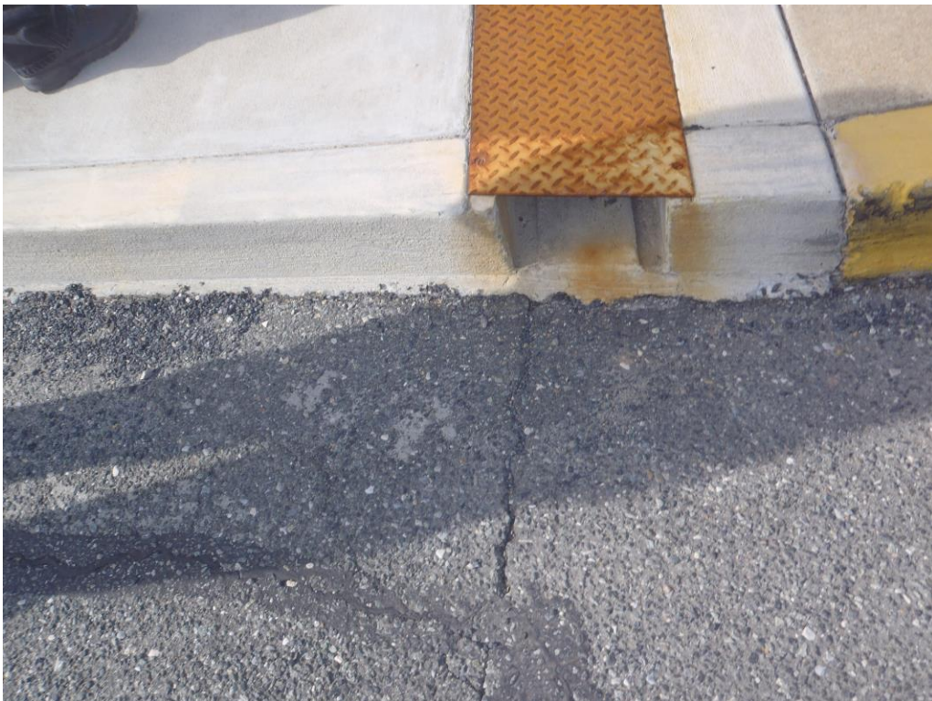
Concrete walk with covered swale for rain leader.
