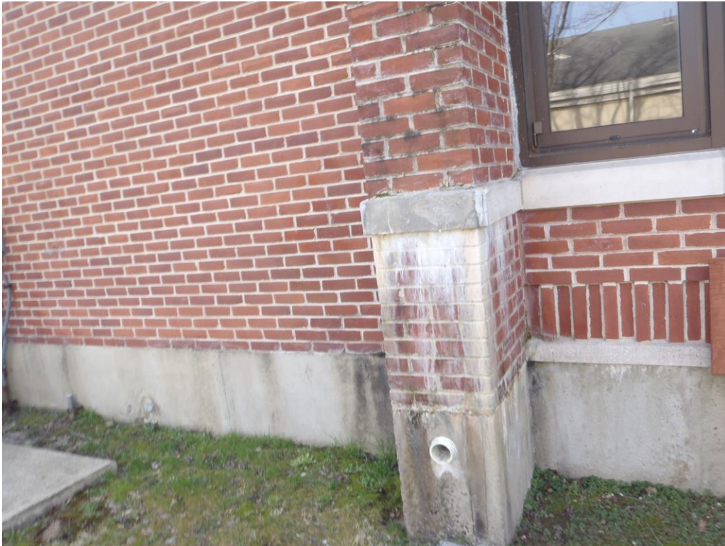
Soluble salts resulting from saturation of mortar of extended periods.
