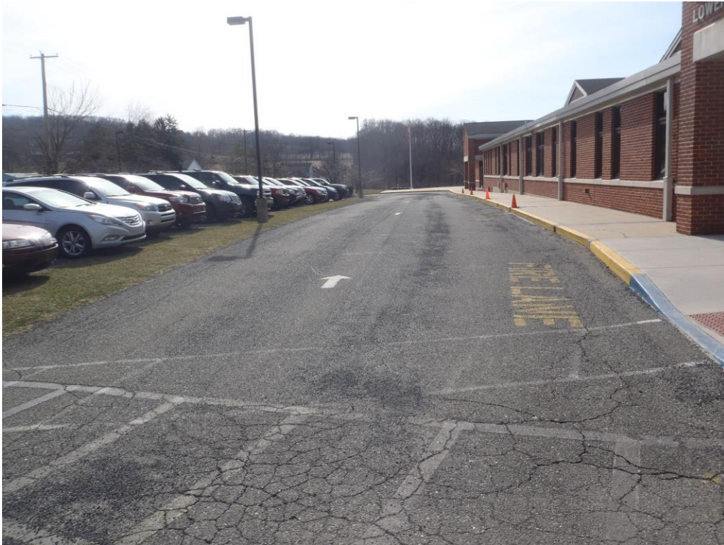
Asphalt paving, typical. Note the extensive alligator cracking.
