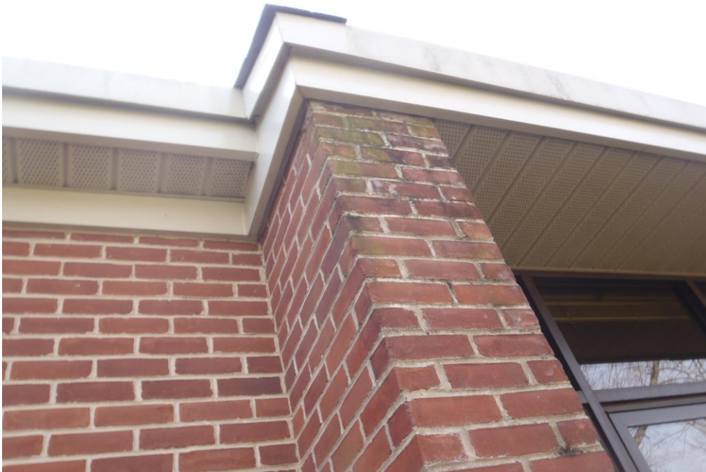
Masonry in area between wings exhibiting staining/loss of mortar resulting from excessive time between drying.
