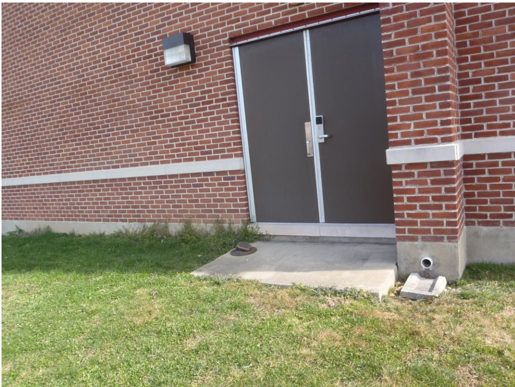
Side entrance. Note the step which limits accessibility.
